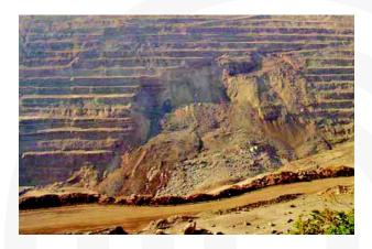
Nchanga Open Pit (NOP) uses SSR technology to optimise safety and recovery In December 2003 a change in movement patterns occurred. Rates temporarily increased to 20mm/day or more in association with blasting and threshold rates increased to between 5 and 10mm/day. In April 2004, instantaneous rate associated with blasting exceeded 150mm/day and the threshold rate increased to 35mm/day.
