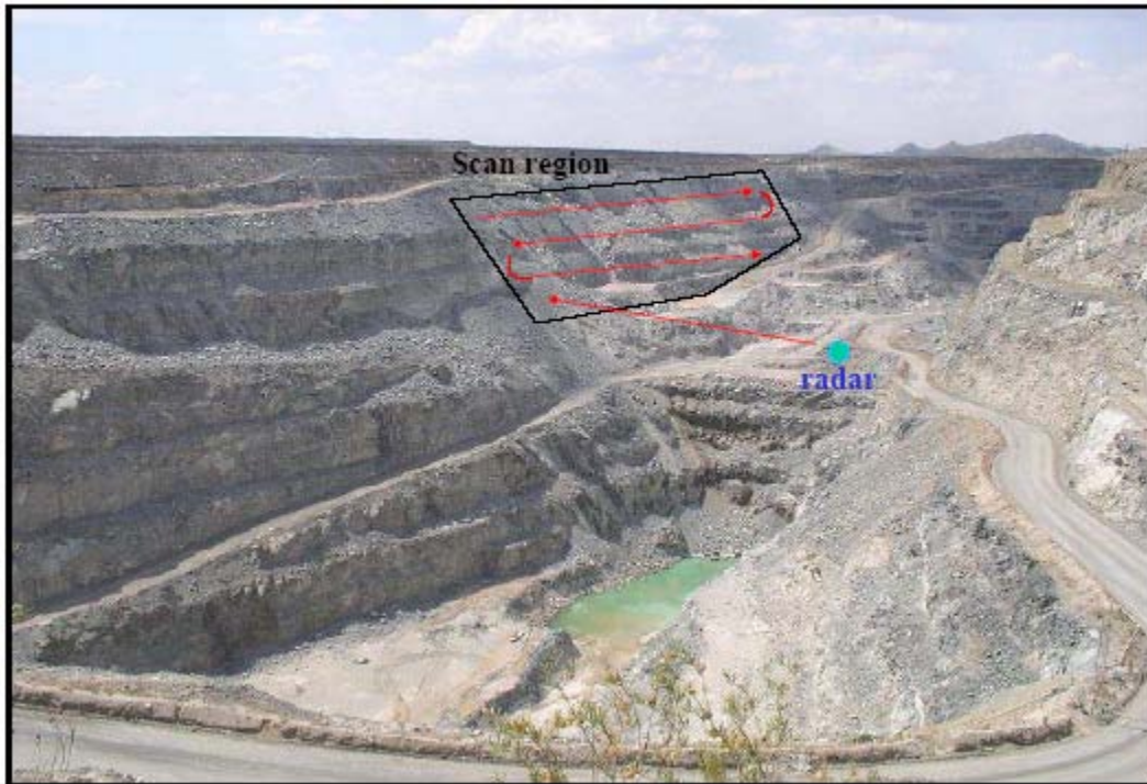
Figure 9 An example of the radar setup in Sandsloot open pit
