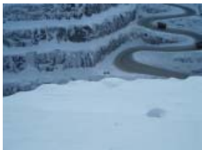
▲ Road down into the pit
